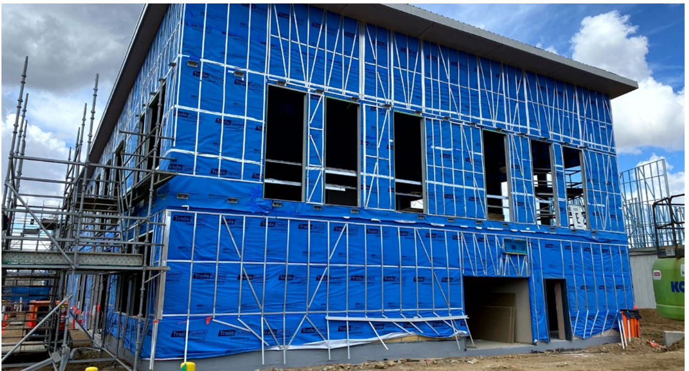
Figure 2: Image of site construction 27 September 2023
