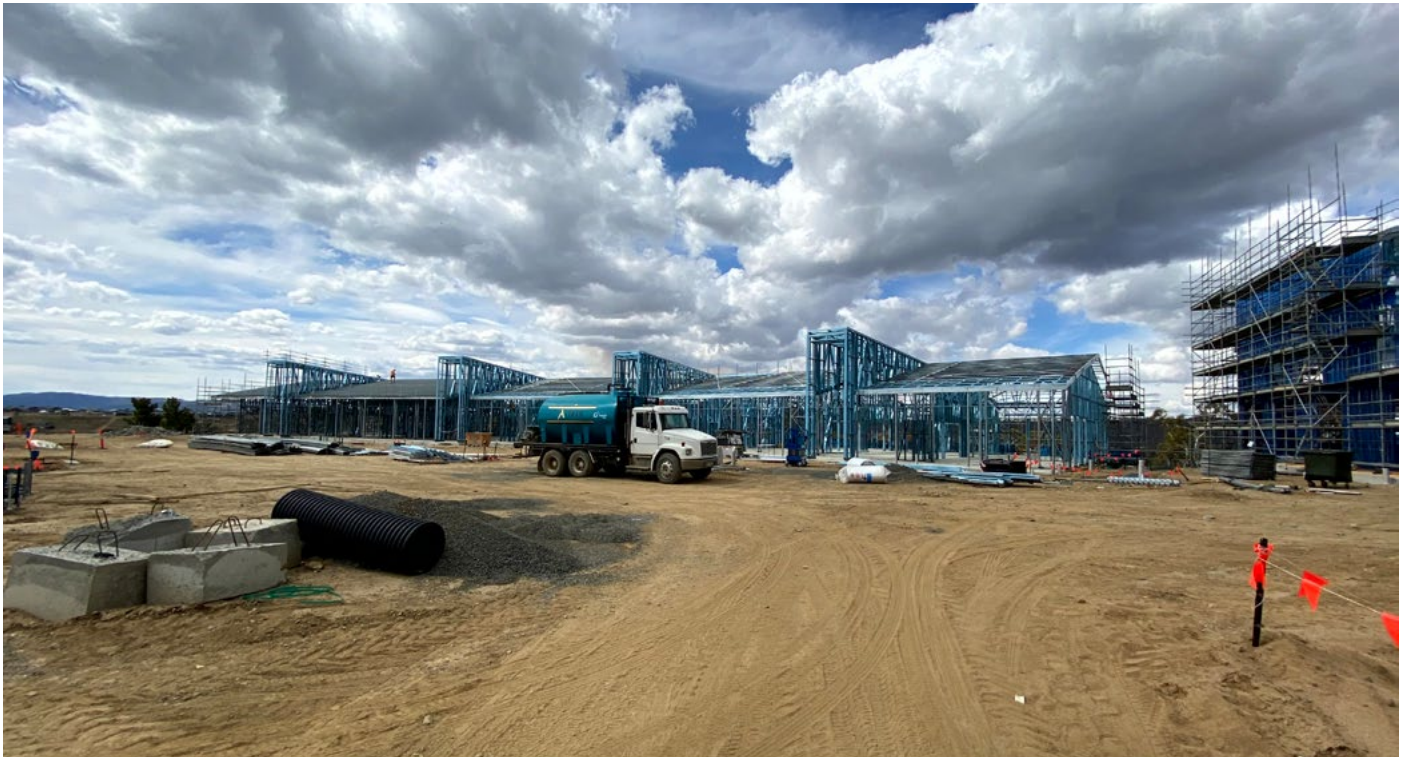
Figure 1: Image of site construction 27 September 2023
