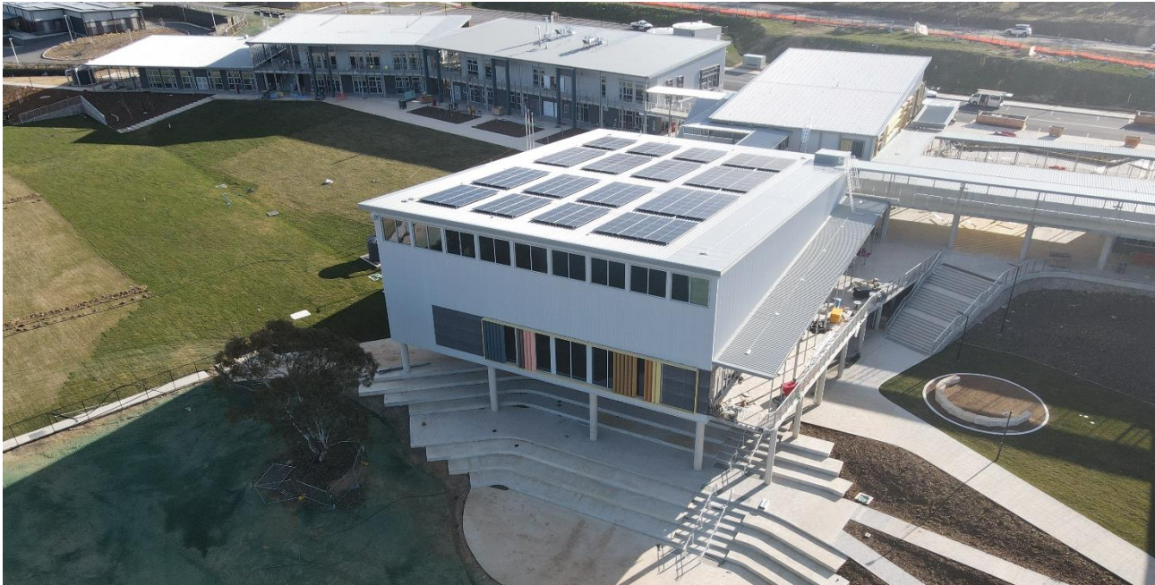
High School gym, amphitheatre, yarning circle and part of the new playground
